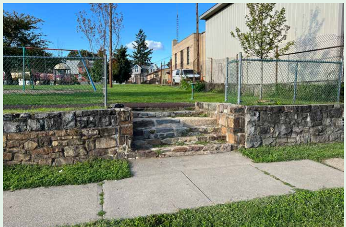
Existing southeast entrance.
